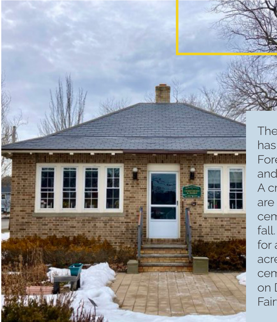
Pictured: The Cemeteries Office building with new roof replacement
